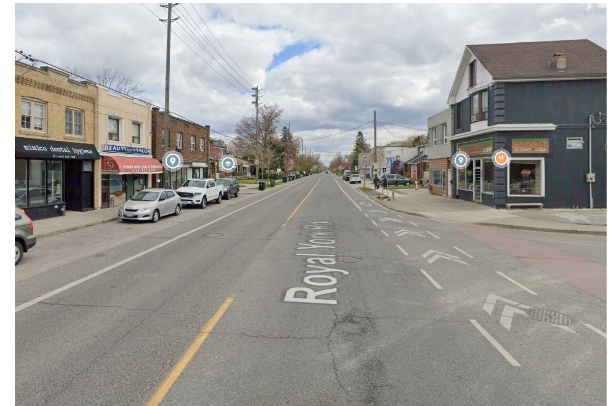
Royal York Road Two traffic lanes, bike lanes, and some parking lay-bys on either side of the street
