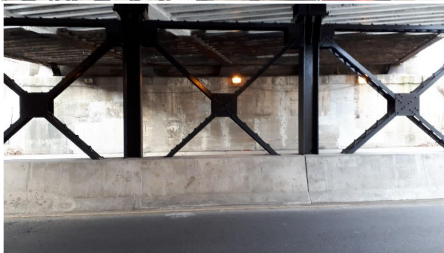
Plate 14: View of "X" bracing and concrete wheel guard.
