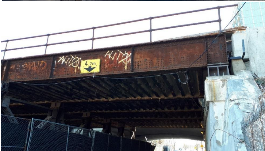
Plate 48: Detail of bridge bearing and handrail.
