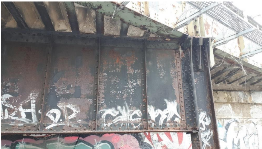
Plate 88: Detail of riveted connections.
