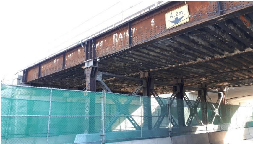
Plate 30: Detail of "X" bracing and bridge bearings on top of bracing.
