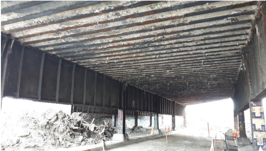
Plate 90: Detail of longitudinal steel beams.
