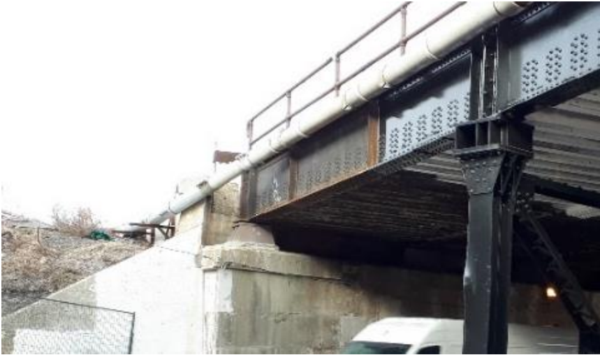
Plate 16: Detail of bridge bearings.
