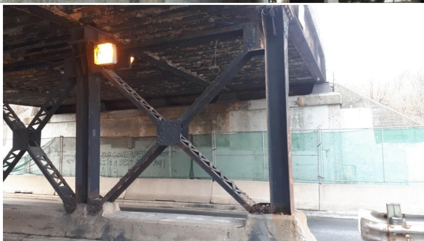
Plate 72: Detail of "X" bracing and western abutment.
