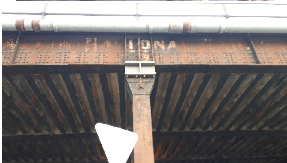
Plate 73: Detail of bearing on top of bracing.
