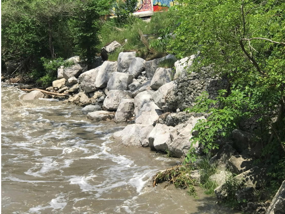
Photograph 3: Close up view existing Gabion Basket wall and Rip-Rap at the toe of the embankment Slope transitioning north (away from the embankment)
