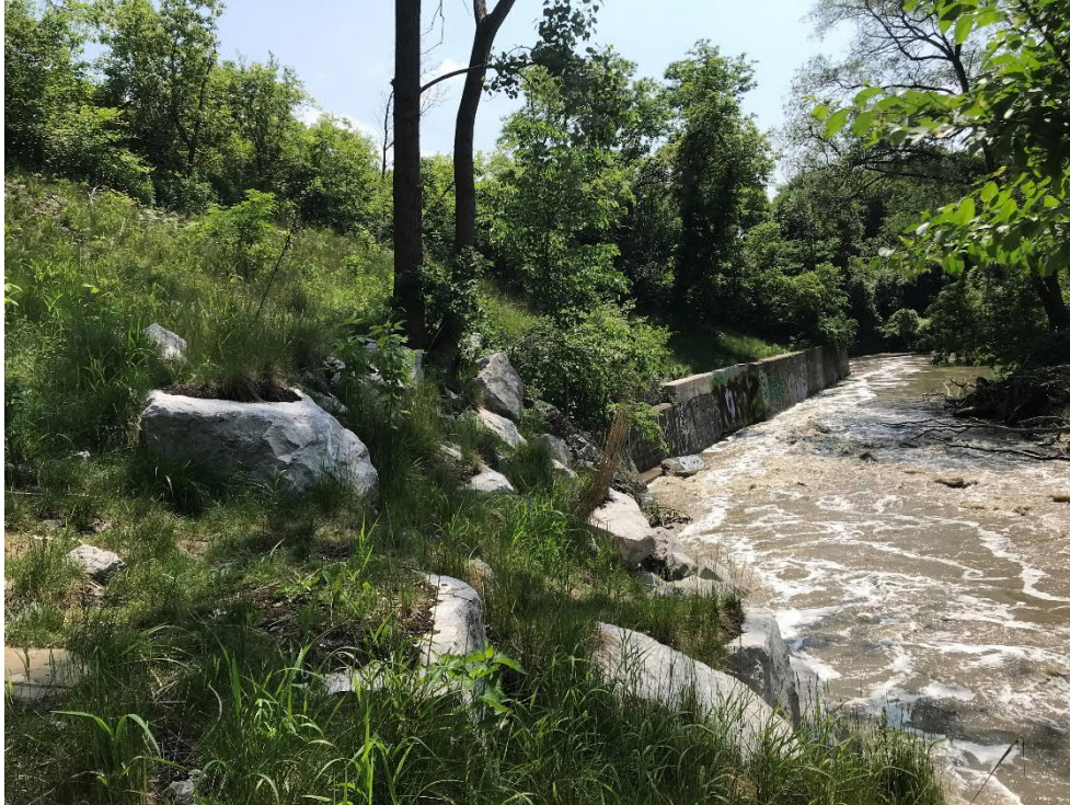
Photograph 1: View of Existing Erosion Protection measures and retaining wall at the toe of the embankment slope at the west end of the site (Looking West towards Mimico Creek Bridge).
