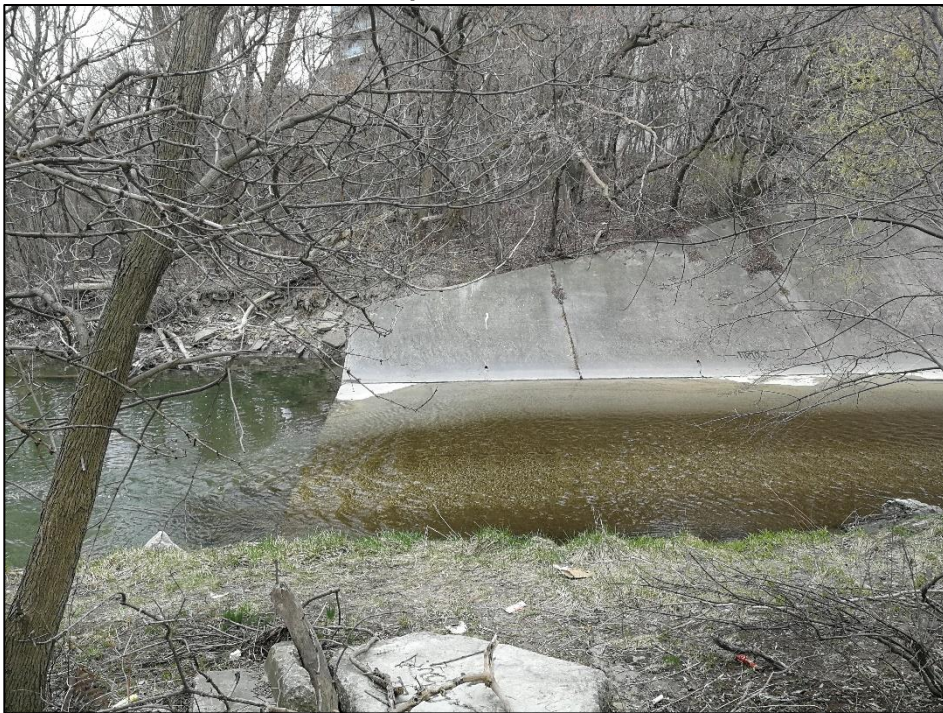
Photograph B-12: View of the potential fish barrier at the downstream end of the concrete channel beneath the Gardiner Expressway (Unit 1), April 17, 2020
