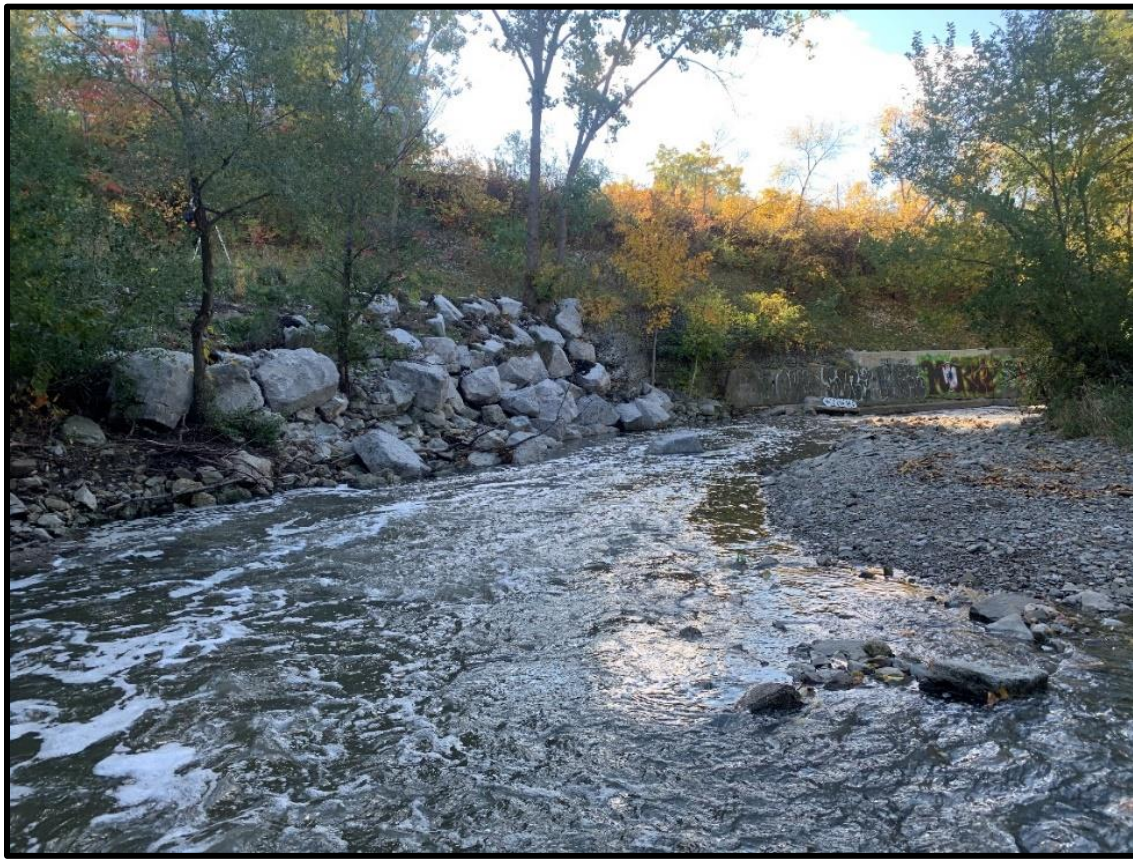
Figure 3: Looking downstream at the armoured bank. Slumping armourstone protects the bend, and the gabion basket and concrete retaining walls can be seen protecting the slope. Note that there are scour pools directly adjacent to the concrete wall.
