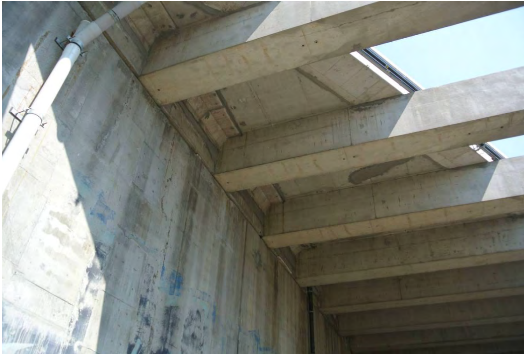
Figure 21: Detail of the concrete beams supporting the bridge deck.
