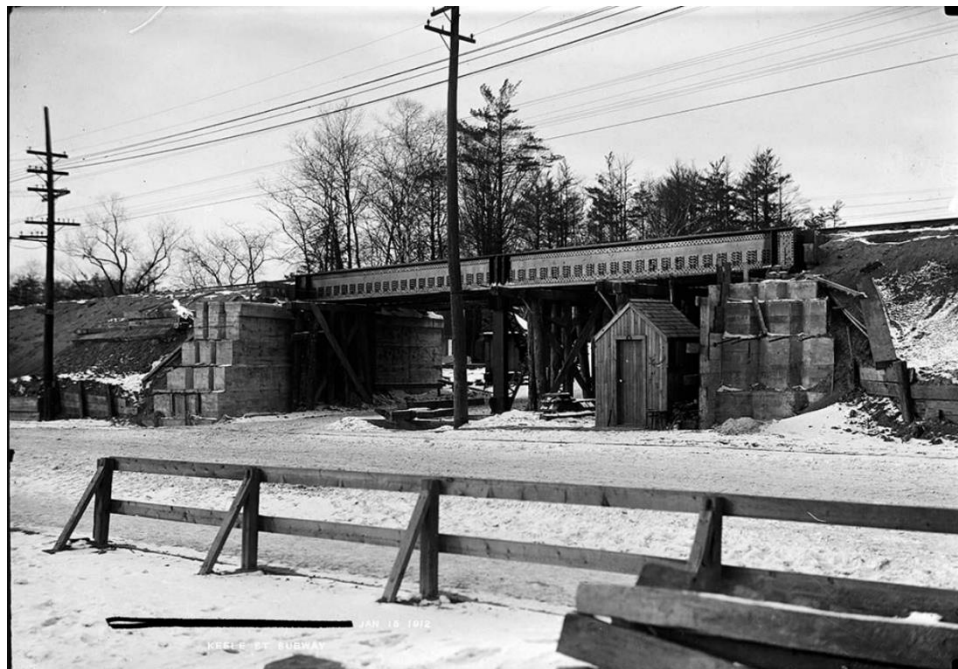
Figure 15: Photograph showing rail crossing Parkside Drive in 1912 (Salmon 1912).
