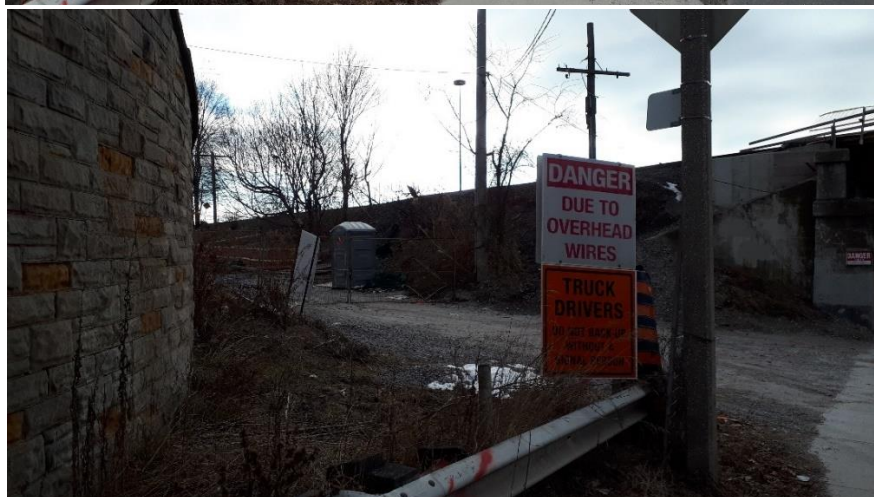
Plate 6: View of the area adjacent to the north of the bridge on the eastern side, looking southeast.
