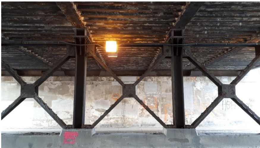
Plate 58: Detail of "X" bracing, bearings, and steel beams.
