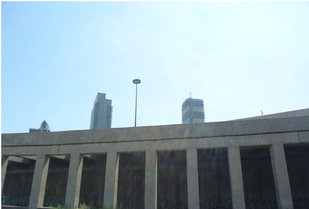
Figure 25: View toward the replaced light standard on the subject bridge.
