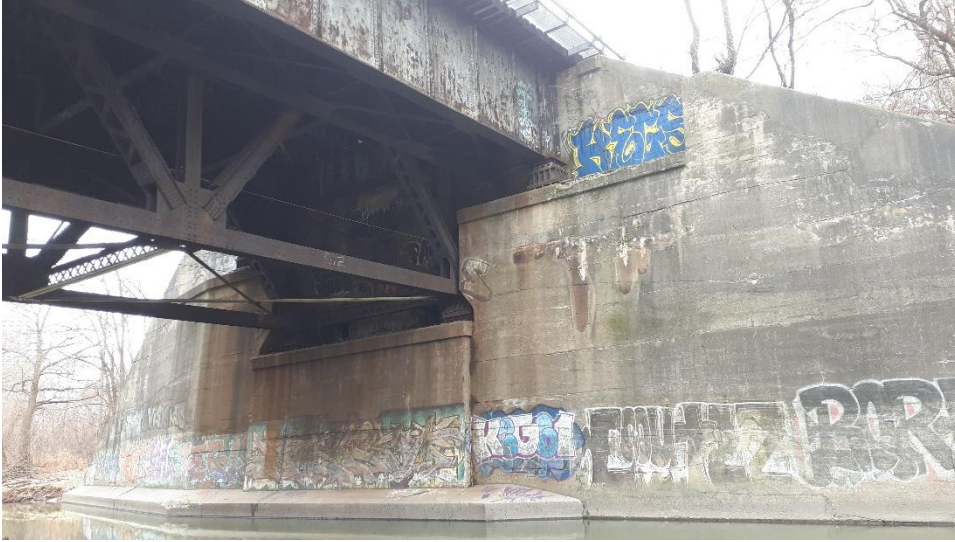
Plate 104: View of east abutment from the south.
