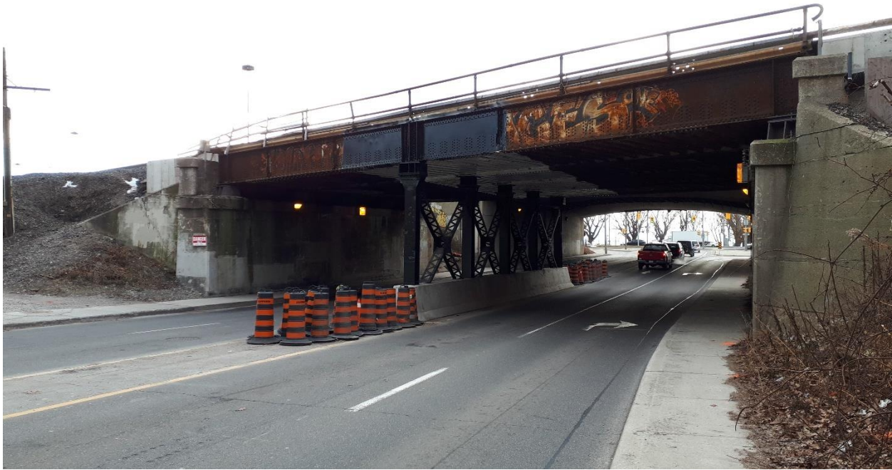
Figure 2: Parkside Drive Bridge (Mile 3.89), facing southeast.
