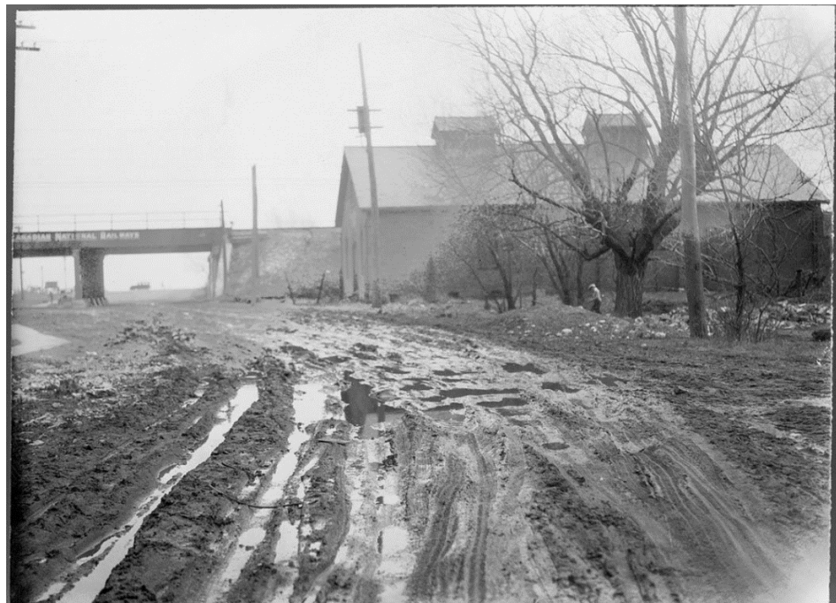
Figure 24: Photograph likely showing rail bridge over Ellis Avenue (N.A. 1928).
