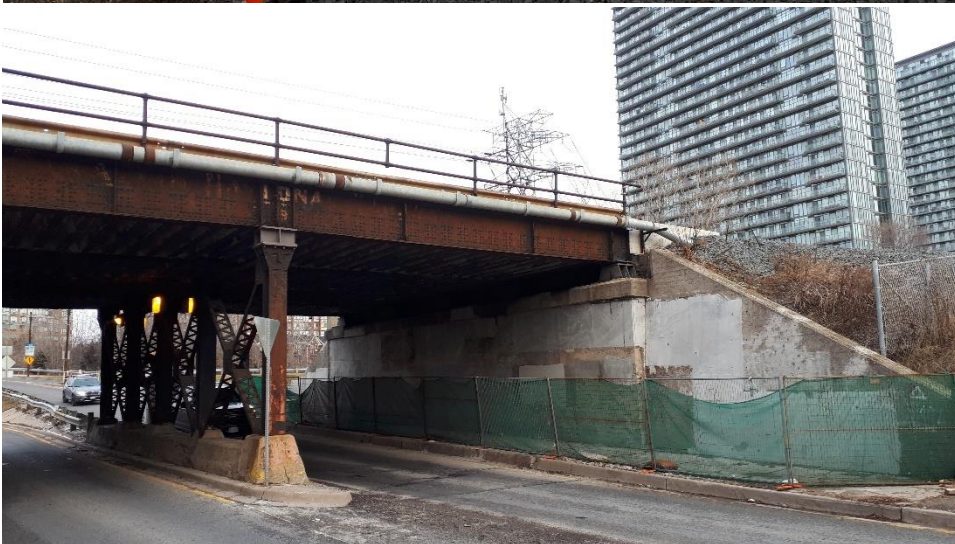
Plate 79: Eastern bridge abutment.
