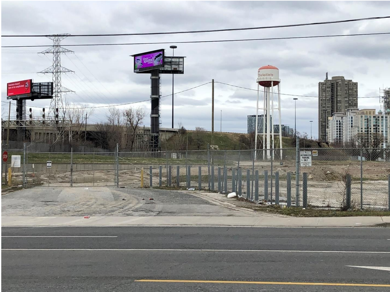
Looking east towards the water tower on the former Mr. Christie Factory site.
