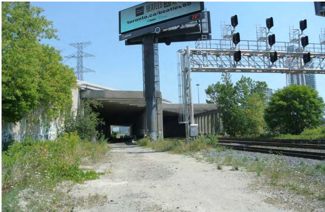
Figure 2: South elevation of the Gardiner Street Bridge.
