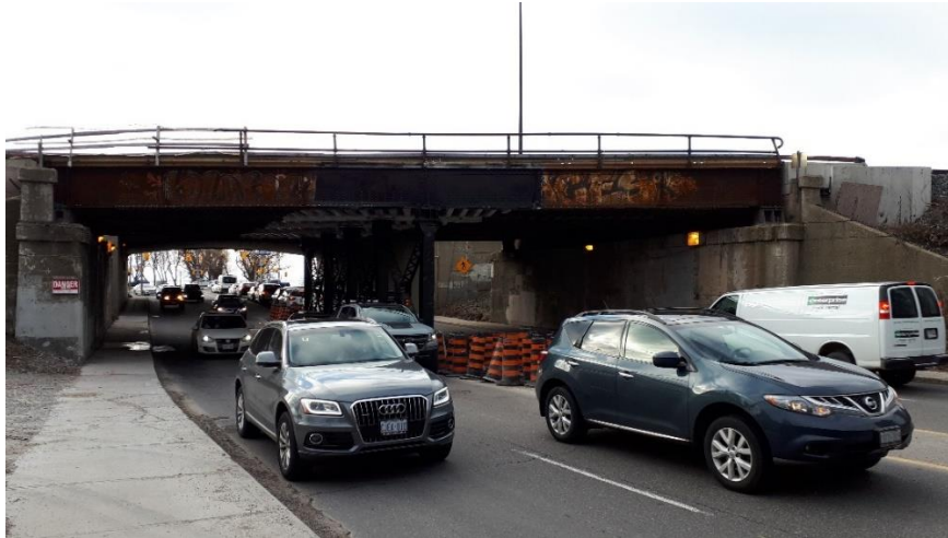
Plate 4: Parkside Drive Bridge (Mile 3.89) northern elevation, looking south southwest.
