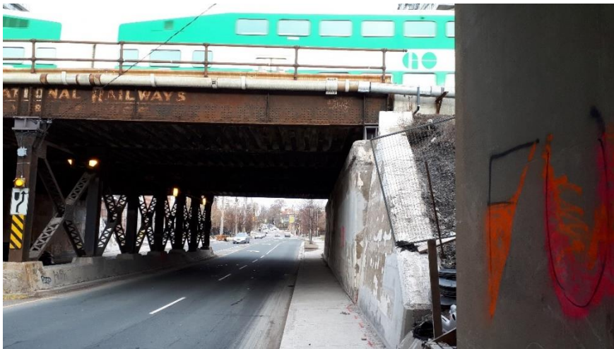
Plate 61: Eastern bridge abutment, looking north.
