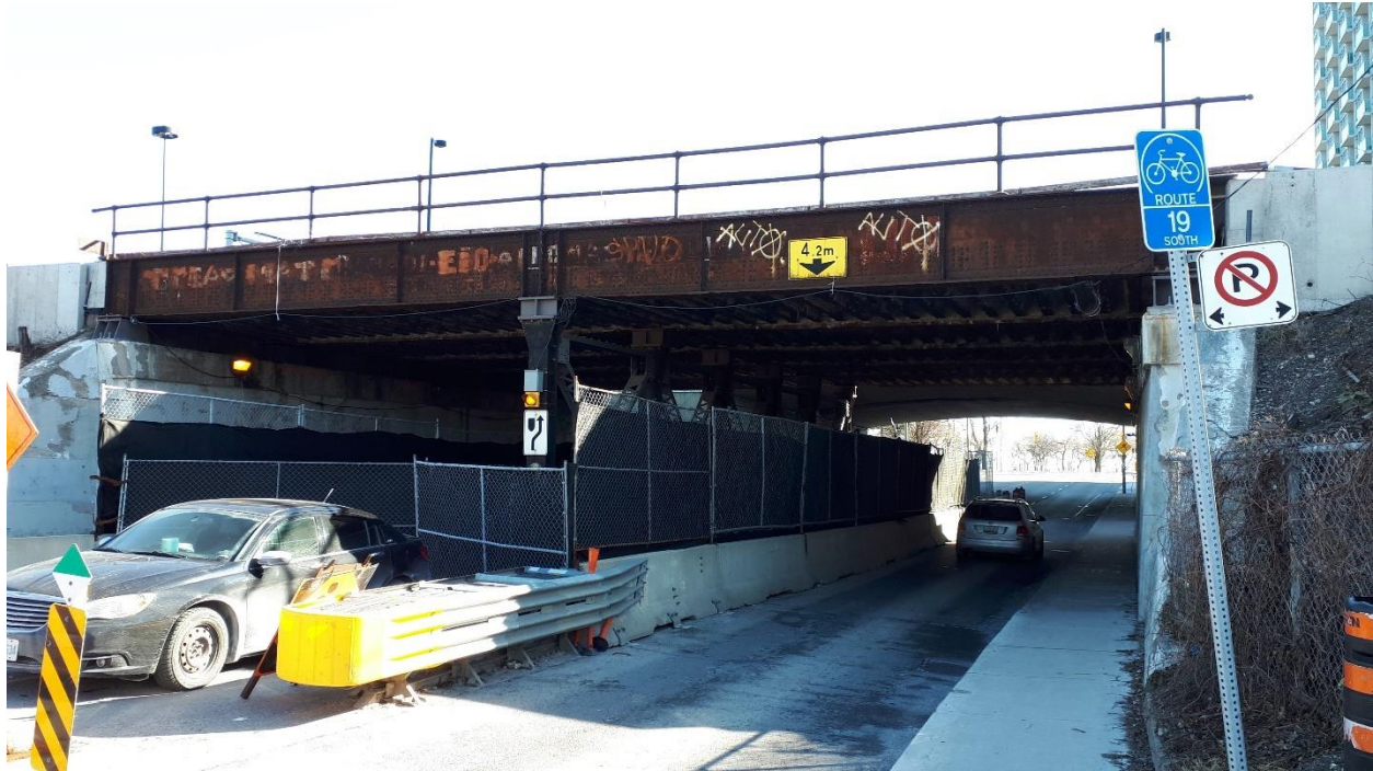
Figure 4: Ellis Avenue Bridge (Mile 4.54), facing southwest.
