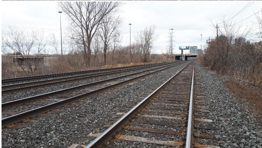
Plate 97: Rail line, looking west.
