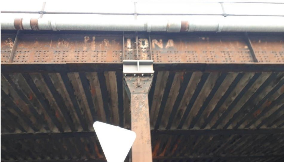
Plate 73: Detail of bearing on top of bracing.
