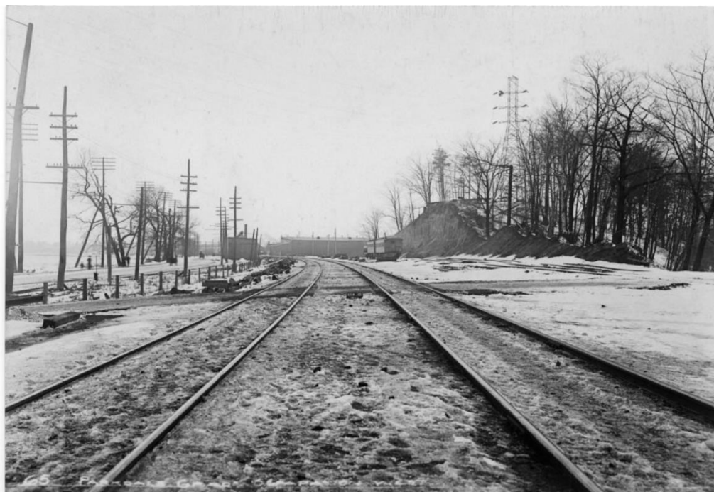
Figure 21: Photograph showing railway at Colborne Lodge Drive (N.A. 1911).
