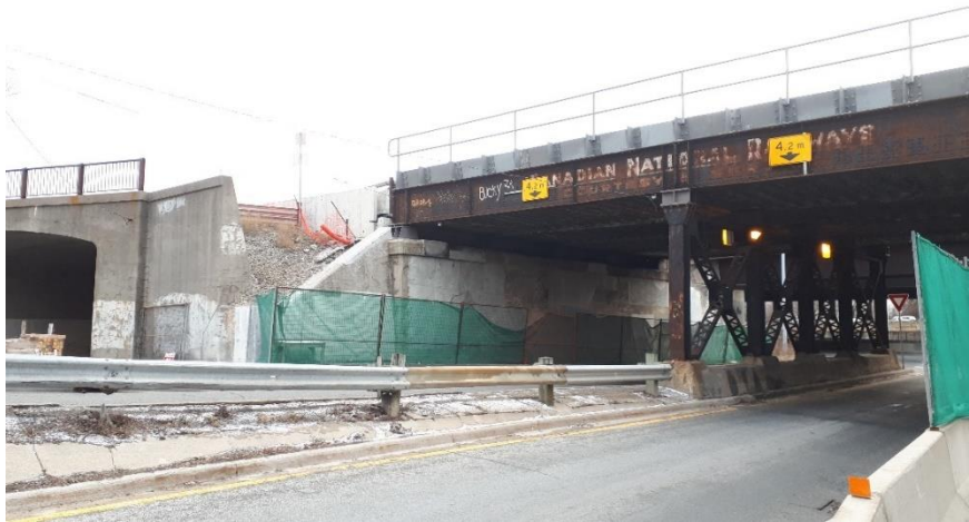
Plate 80: Western bridge abutment.
