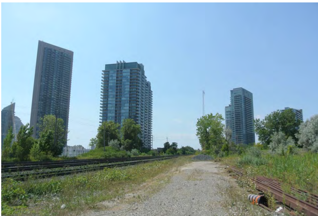
Figure 26: View of the railway corridor approaching the bridge to the west, looking west.
