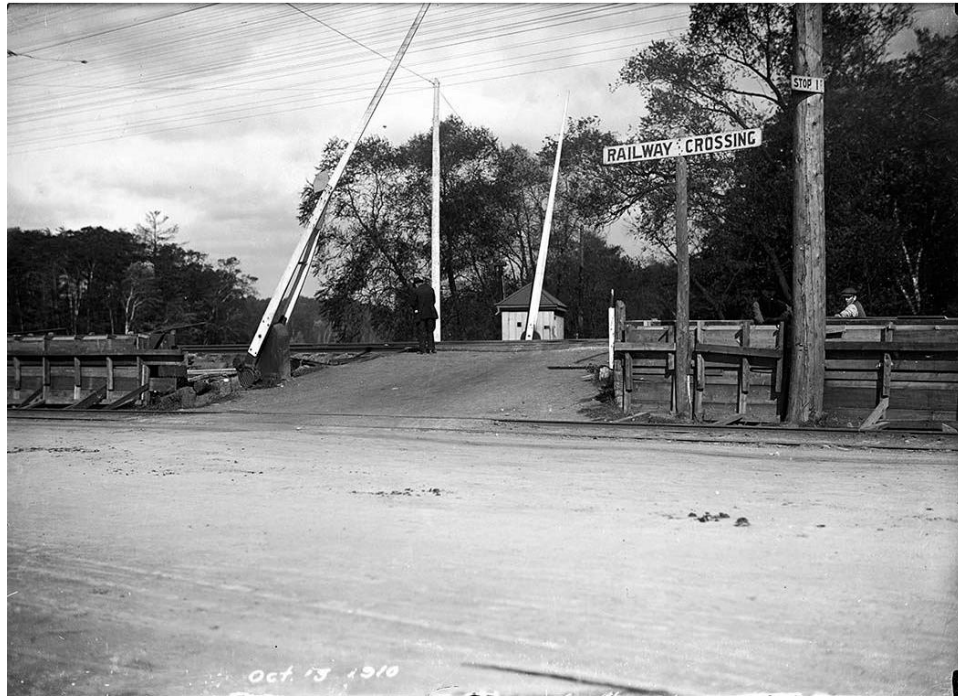
Figure 14: Photograph showing rail crossing at Parkside Drive in 1910 (Salmon 1910a).
