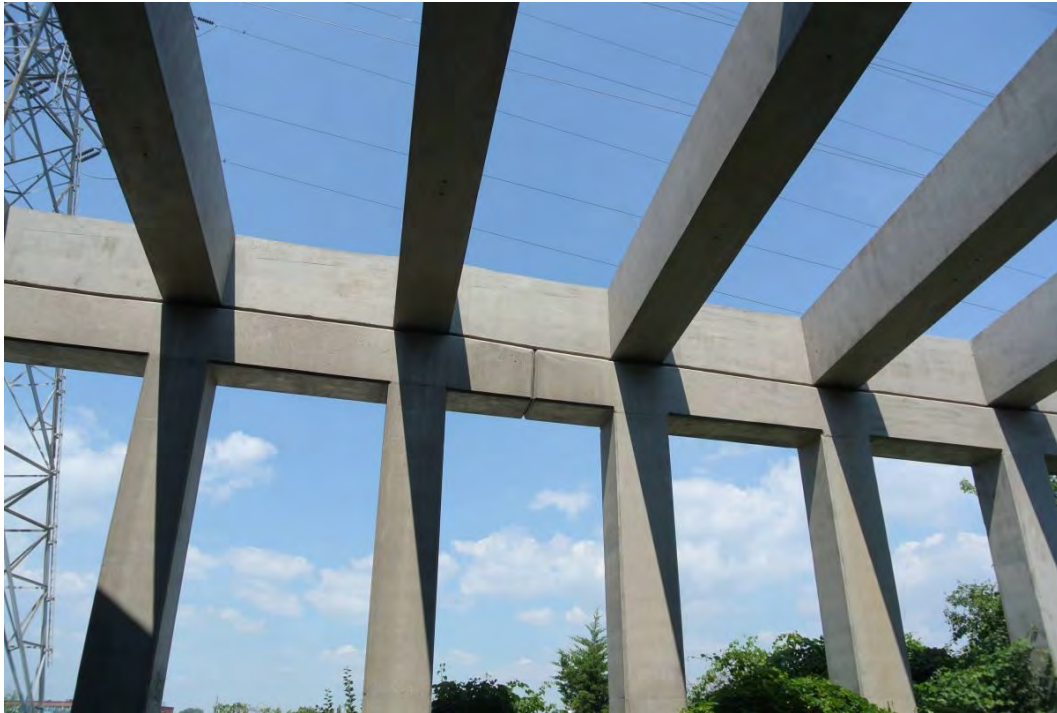
Figure 19: View of columns extending from northwest abutment, looking north.
