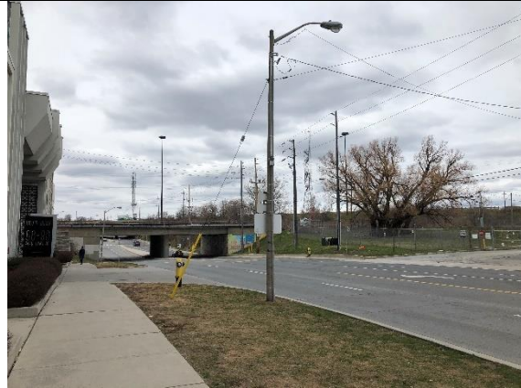
Plate 1: View north along Park Lawn Road towards rail corridor.
