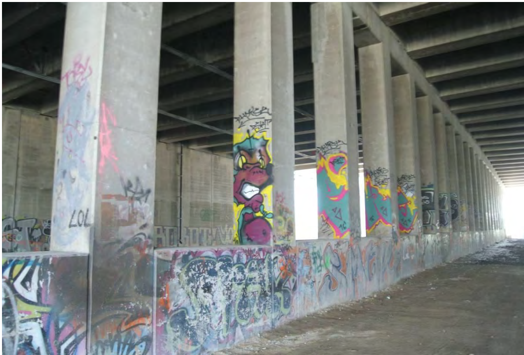
Figure 23: View of concrete columns comprising the single pier, looking west.
