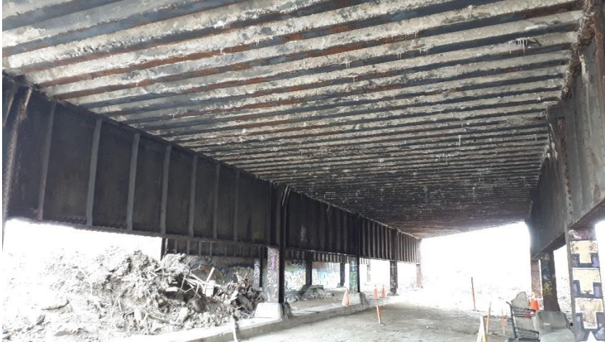
Plate 90: Detail of longitudinal steel beams.
