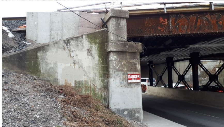
Plate 8: Eastern bridge abutment, looking south.
