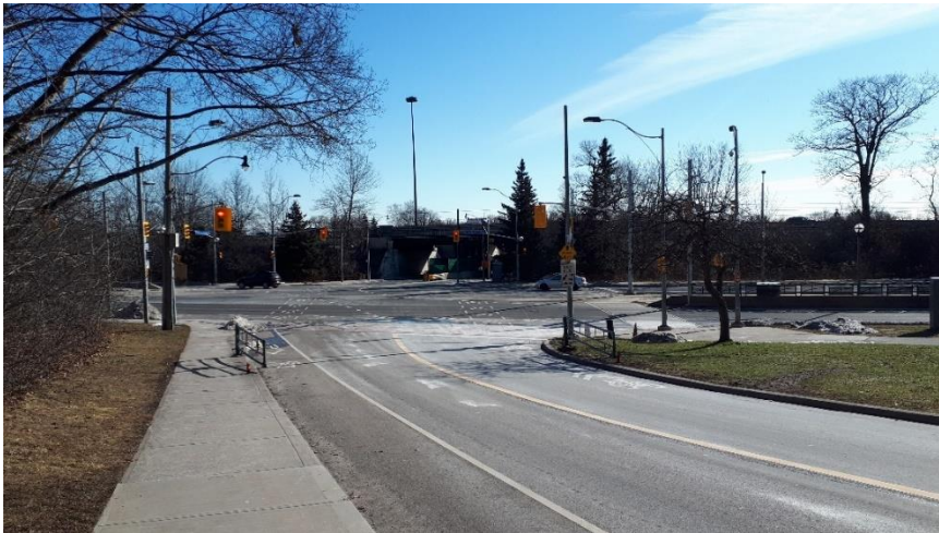
Plate 25: Colborne Lodge Drive and the Queensway north of the bridge, looking southeast.
