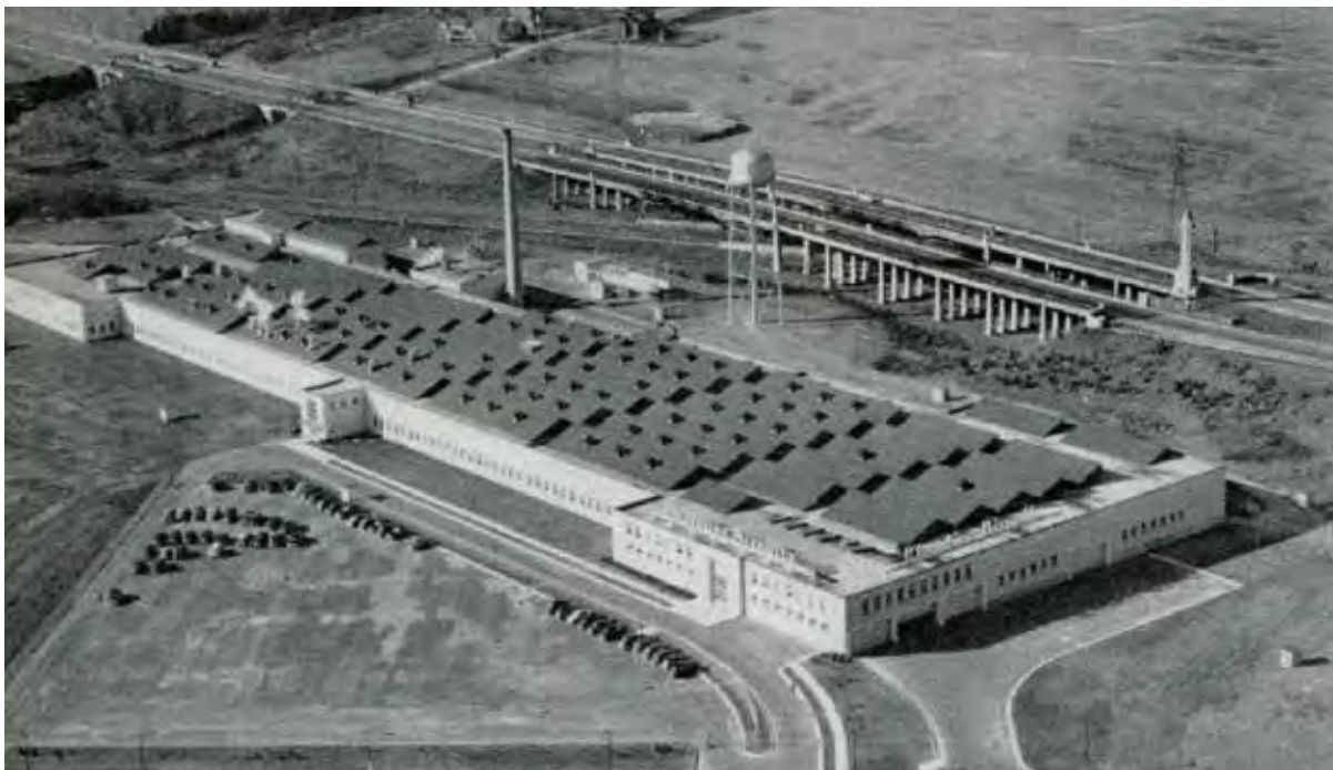
Aerial photograph of the Lakeshore Bakery (RAIC Journal, Feb 1950).
