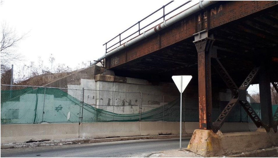
Plate 77: Western bridge abutment, looking northwest.
