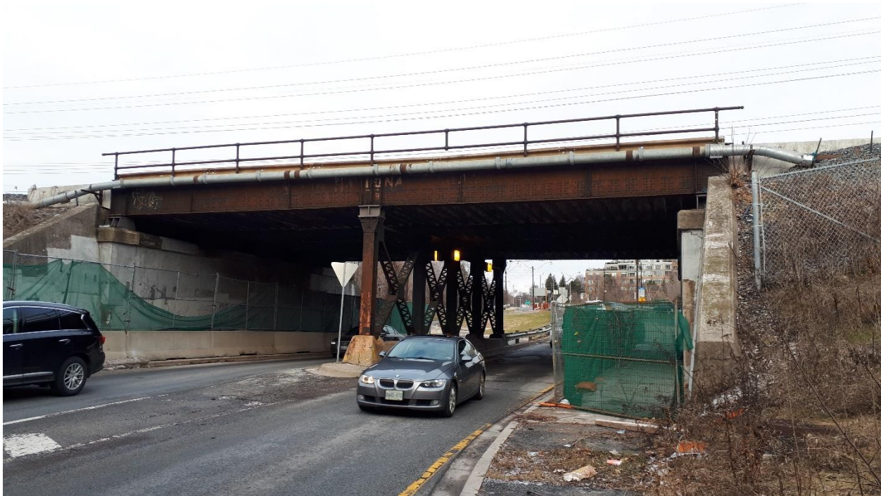
Figure 6: Gardiner On-Ramp from Riverside Drive (Mile 4.90), facing northwest.
