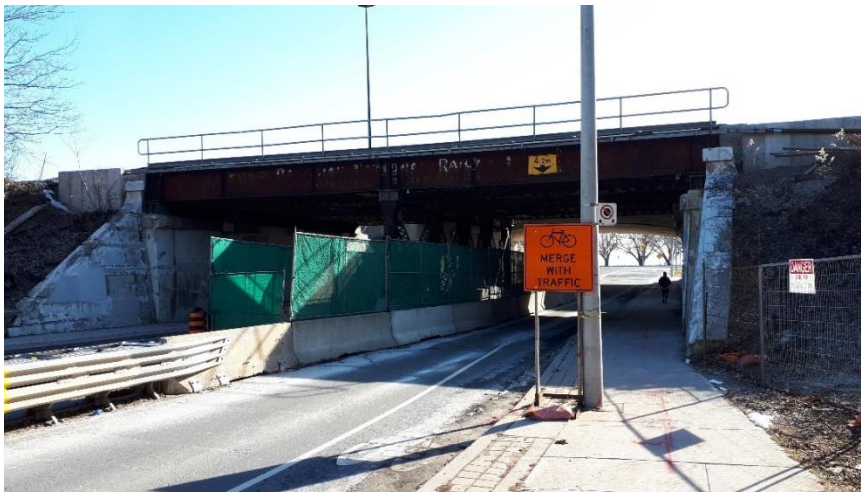
Plate 26: Colborne Lodge Drive Bridge (Mile 4.17) north elevation, looking southeast.
