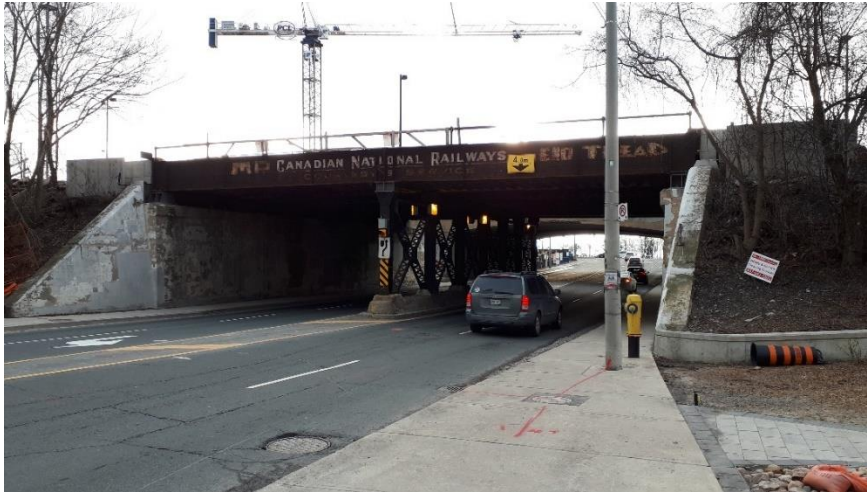
Plate 66: Northern bridge elevation, looking southeast.
