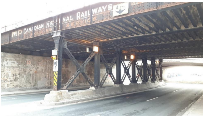
Plate 65: Northern bridge elevation, looking southeast.
