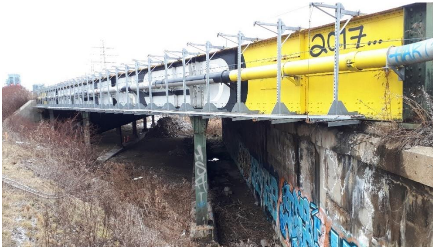
Plate 94: Southern bridge elevation.
