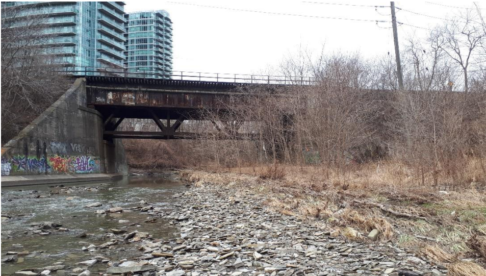
Plate 99: Northern bridge elevation, looking south.
