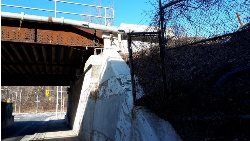
Plate 37: Eastern abutment, looking north.
