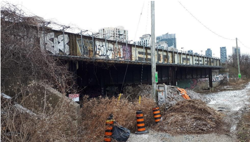
Plate 84: Northern bridge elevation, looking southwest.
