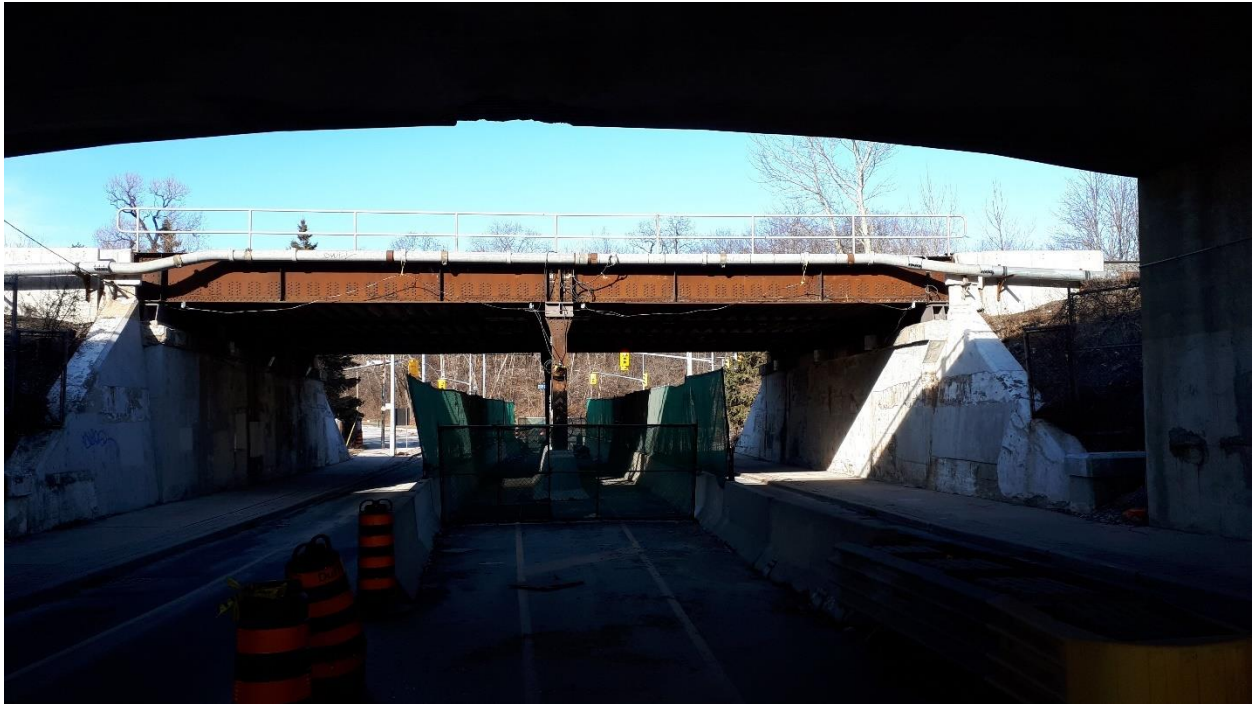
Figure 3: Colborne Lodge Drive Bridge (Mile 4.17), facing north.
