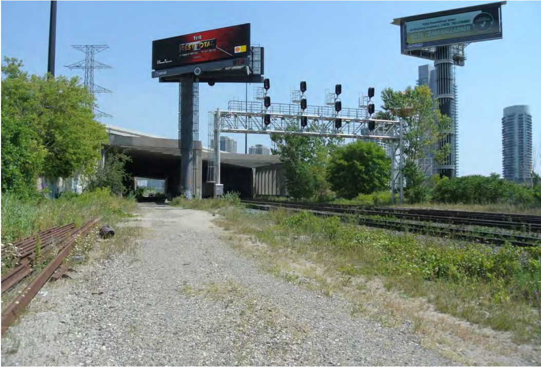
Figure 17: View of west elevation, looking east.
