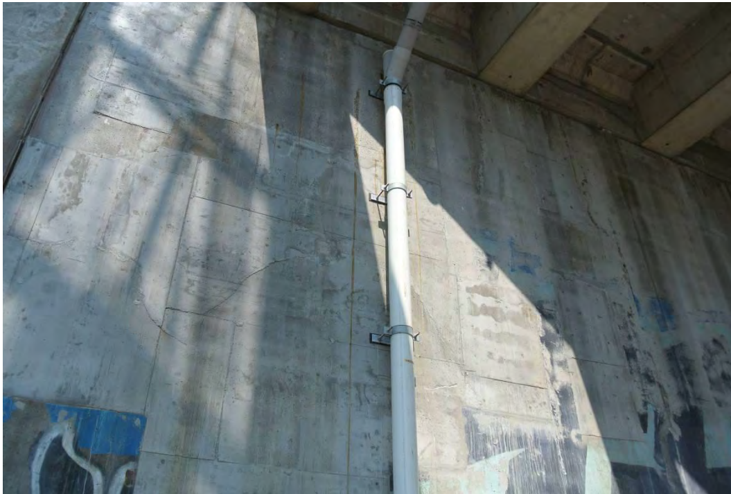
Figure 22: Detail of drainage system on the northwest abutment.
