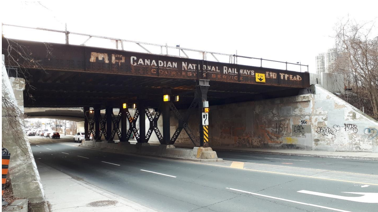
Figure 5: Windermere Avenue Bridge (Mile 4.70), facing southwest.
