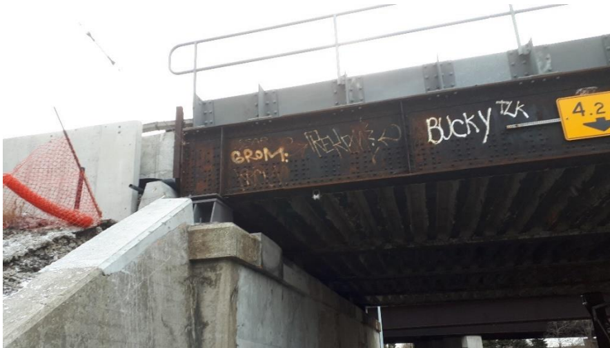
Plate 71: View of bridge bearing and steel handrail.
