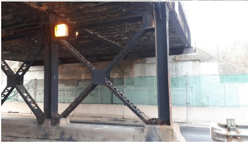
Plate 72: Detail of "X" bracing and western abutment.
