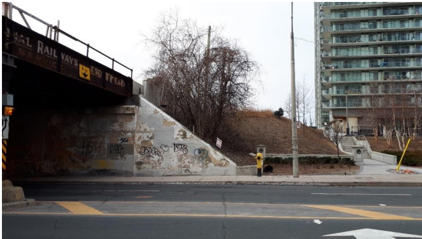
Plate 56: Western bridge abutment, looking west.
