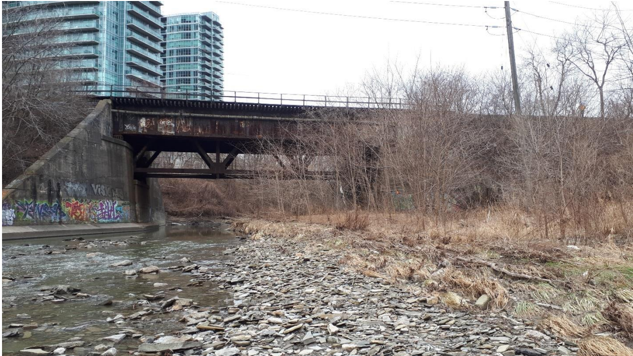
Figure 8: Mimico Creek Bridge (Mile 5.94), facing southeast.
