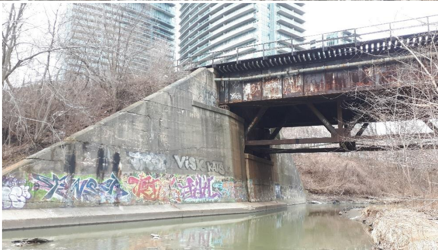
Plate 100: Detail of eastern bridge abutment.
