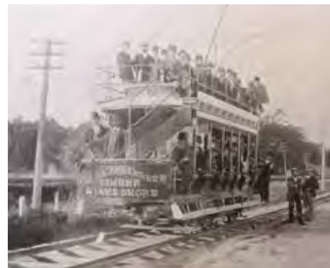
The Toronto & Mimico Electric Railway, later the Toronto & York Radial Railway, enabled easier access to the Site and surroundings from Toronto, and ultimately fostered its residential, recreational and industrial development (Toronto Public Library, c. 1891).
