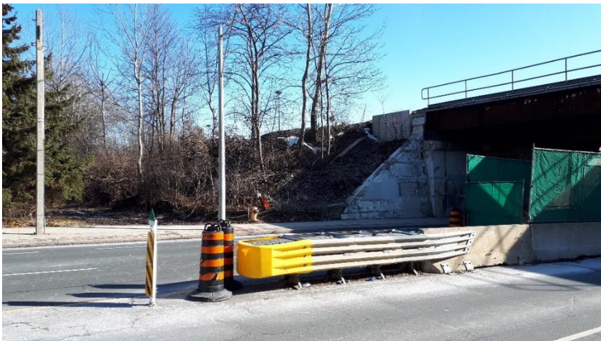
Plate 27: Detail of eastern abutment, looking southeast.
