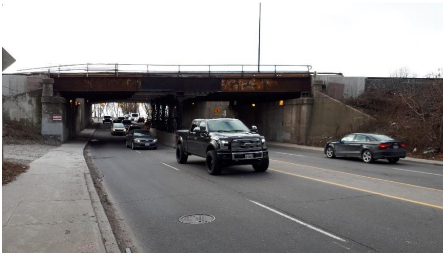
Plate 1: Parkside Drive Bridge (Mile 3.89) north elevation, looking south.
