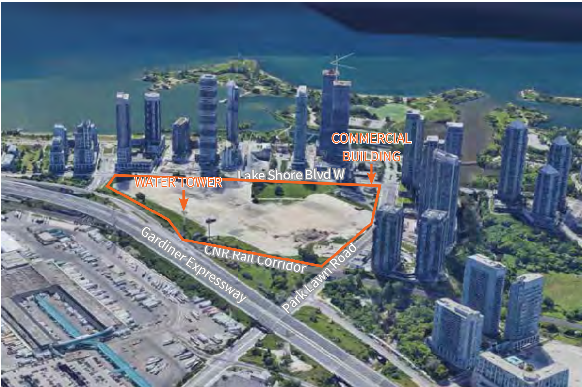
Axonometric view, showing the Site in orange (Google Maps, annotated by ERA).
