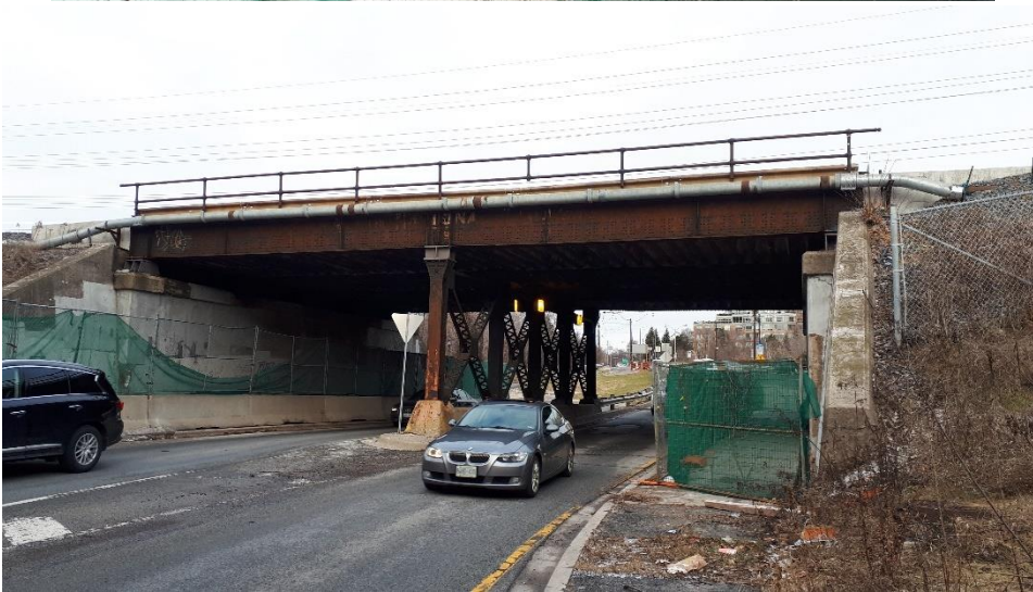
Plate 75: Southern bridge elevation, looking northwest.
