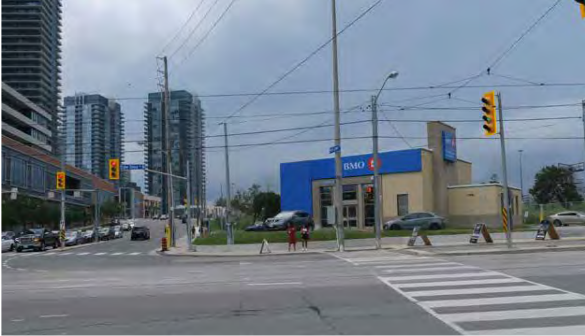
Northward view from the corner of Park Lawn and Lake Shore of the bank building on the Site at 2194 Lake Shore Boulevard West (ERA, 2019).
