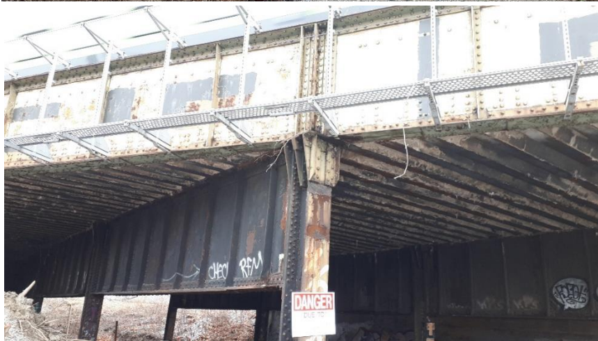
Plate 85: Detail of steel elements.
