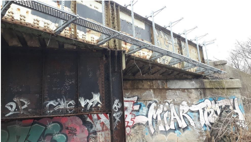
Plate 87: Detail of the bridge on top of the abutment.
