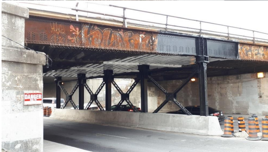
Plate 9: Detail of the steel column and wheel guard, looking west southwest.
