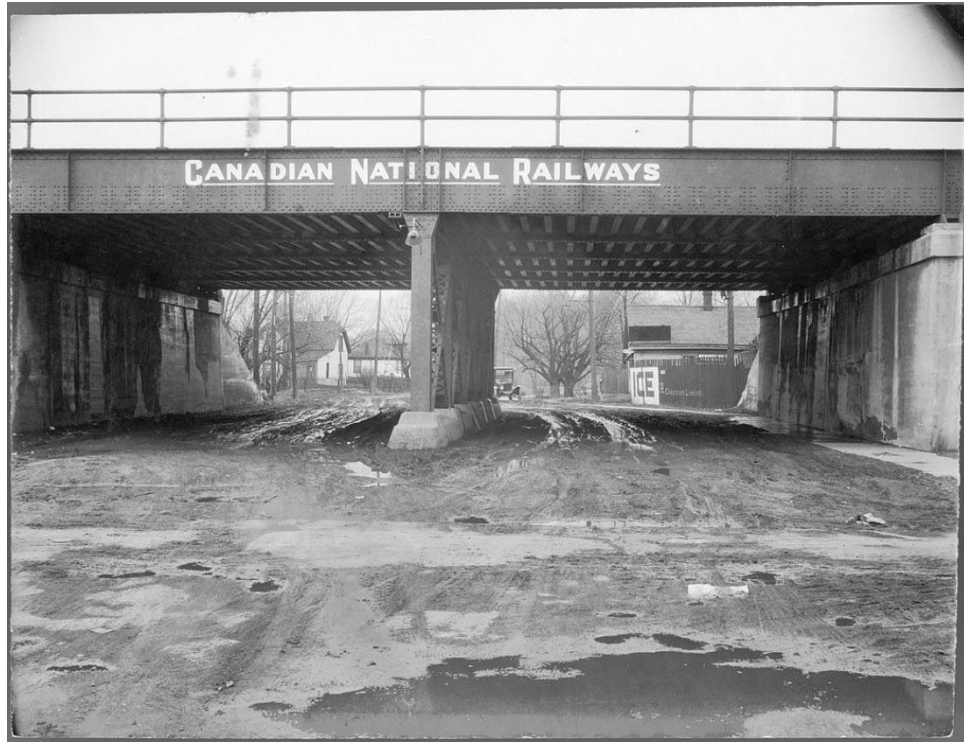
Figure 25: Photograph showing the Ellis Avenue Bridge (Mile 4.54) (N.A. c1928).
