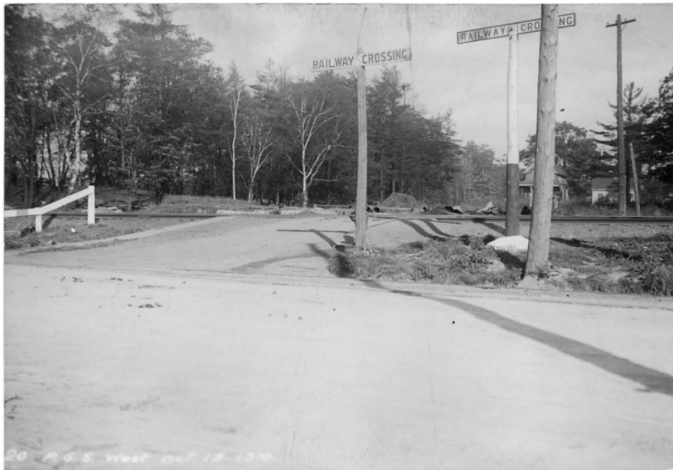
Figure 20: Photograph showing rail crossing at Colborne Lodge Drive (Salmon 1910b).
