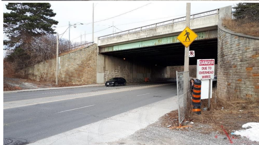
Plate 12: View of the Queensway bridge north of Parkside Drive Bridge (Mile 3.89), looking northwest.
