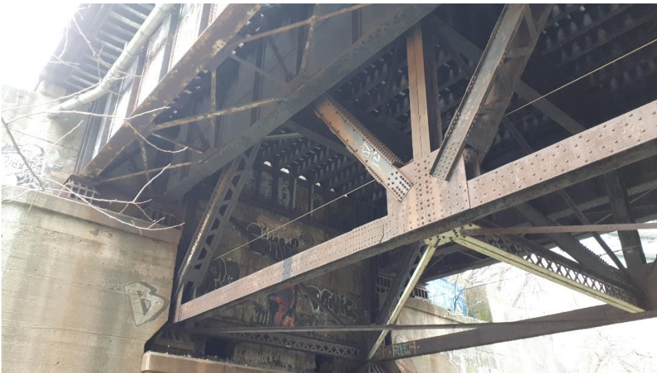
Plate 102: Detail of the bridge superstructures, north side.
