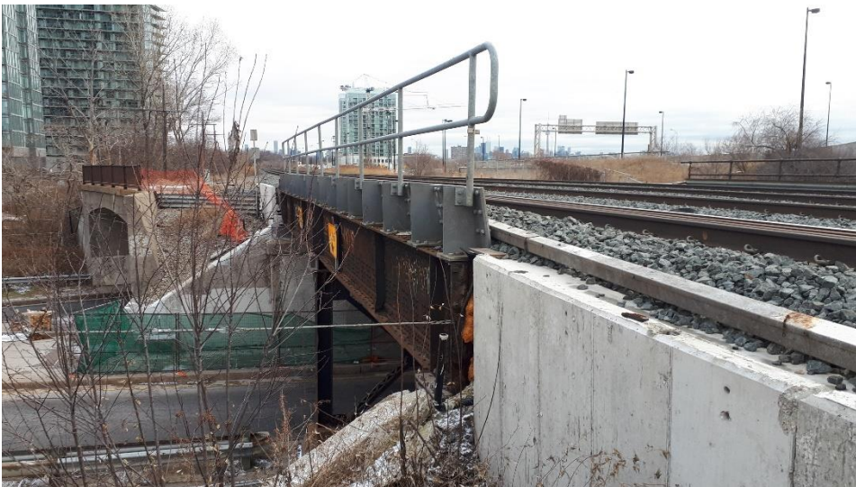
Plate 82: Detail of the steel handrail.
