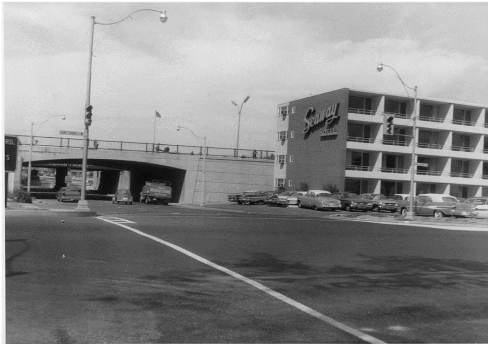
Figure 26: Photograph showing the Windermere Avenue Bridge (Mile 4.70) (N.A. c1960).
