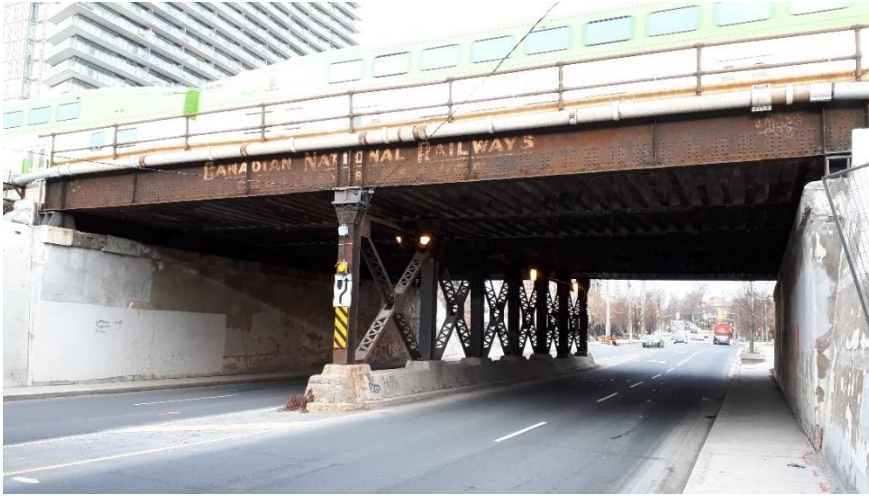
Plate 60: Southern bridge elevation, looking northwest.
