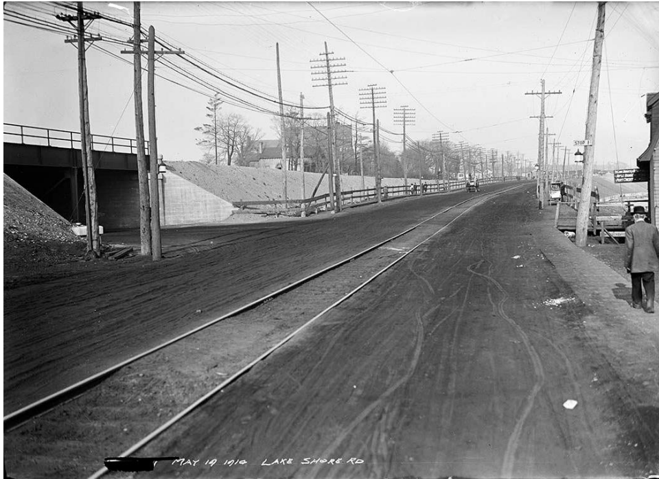
Figure 16: Photograph showing rail crossing Parkside Drive in May 1914 (Salmon 1914a).
