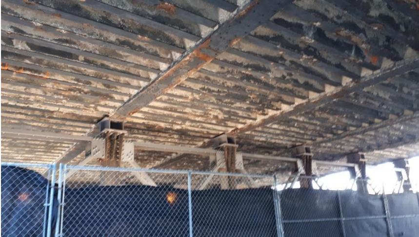
Plate 43: Detail of transverse and longitudinal beams.
