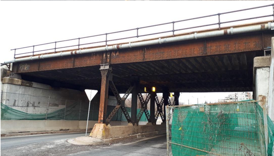
Plate 76: Detail of bracing, concrete wheel guard and median.
