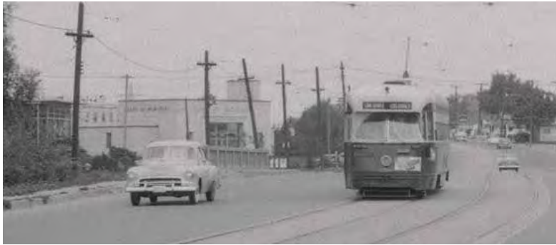
A 1954 view eastward along Lake Shore Boulevard West, with the bank visible in the background behind the car (Toronto Public Library).
