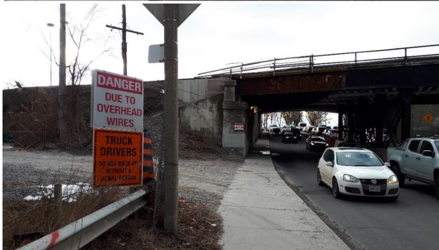
Plate 5: Eastern bridge abutment, looking south.
