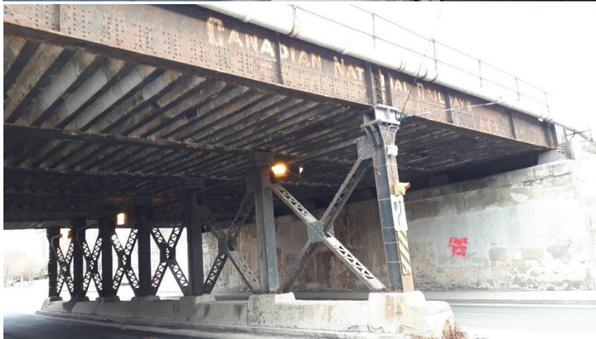
Plate 62: Detail of the bracing and the concrete wheel guard.
