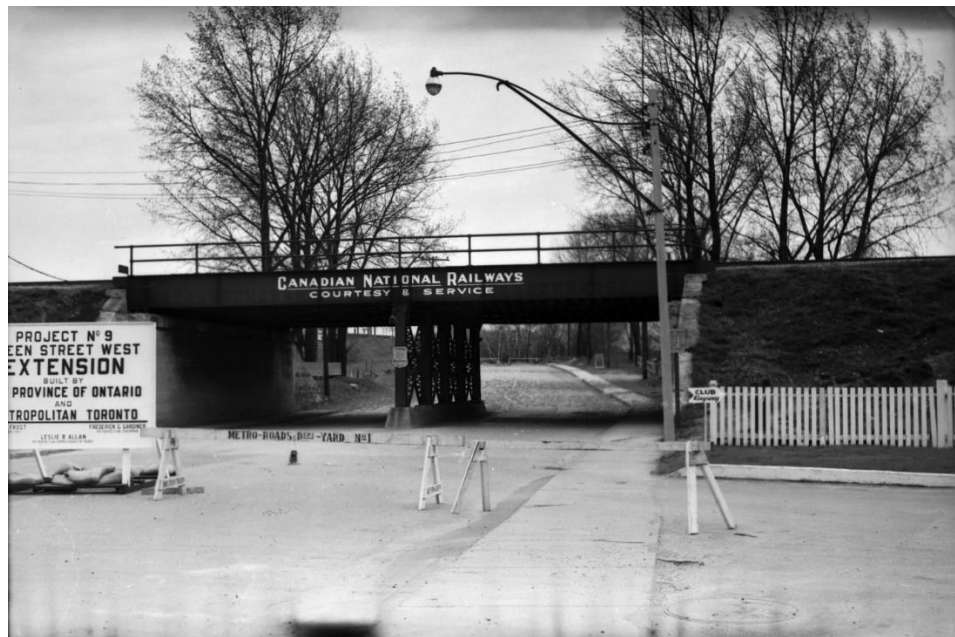
Figure 28: Photograph showing the bridge at the Gardiner On-Ramp from Riverside Drive (Mile 4.90) (Salmon 1955c).
