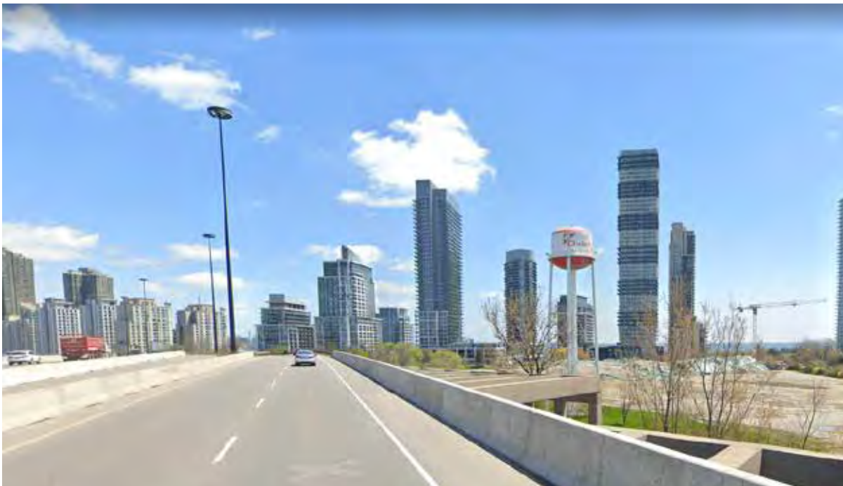
View into the Site (right) while driving eastbound along the Gardiner Expressway (Google Streetview, 2019).
