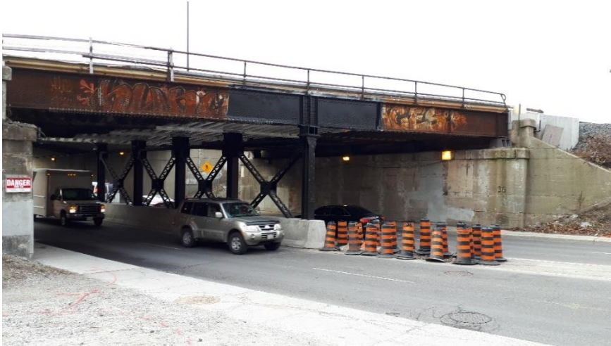
Plate 7: North elevation of Parkside Drive Bridge (Mile 3.89), looking west southwest.
