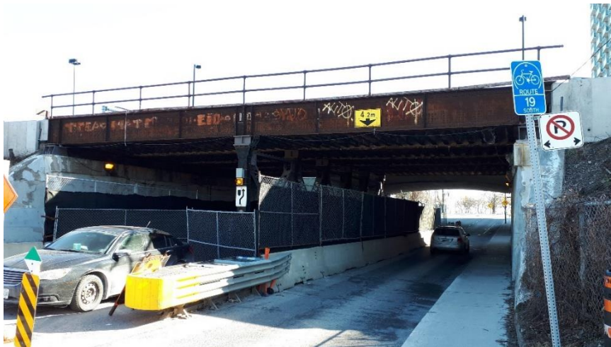
Plate 45: Northern bridge elevation, looking southwest.
