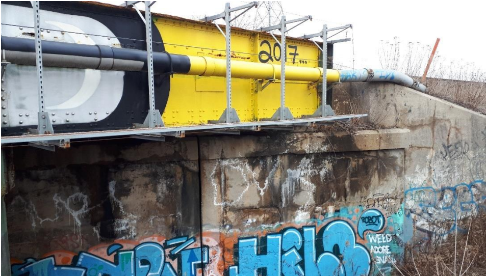
Plate 93: Detail of eastern abutment.
