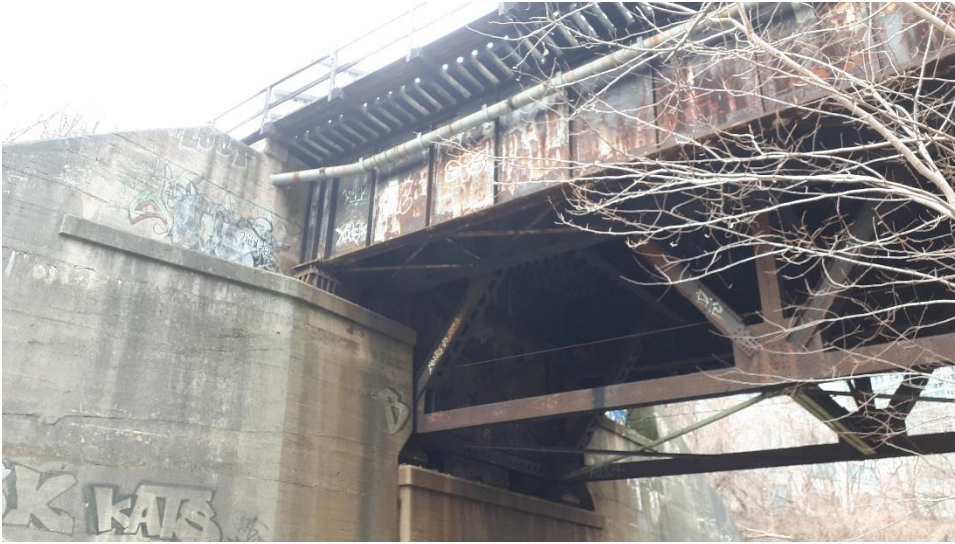
Plate 101: Detail of bridge bearing, east abutment, from the north.
