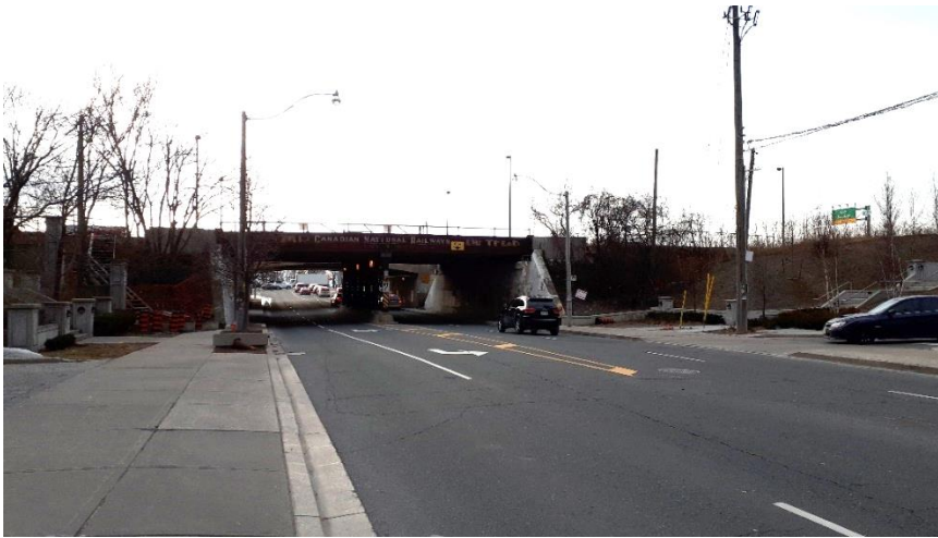
Plate 51: Windermere Avenue north of the bridge, looking south.
