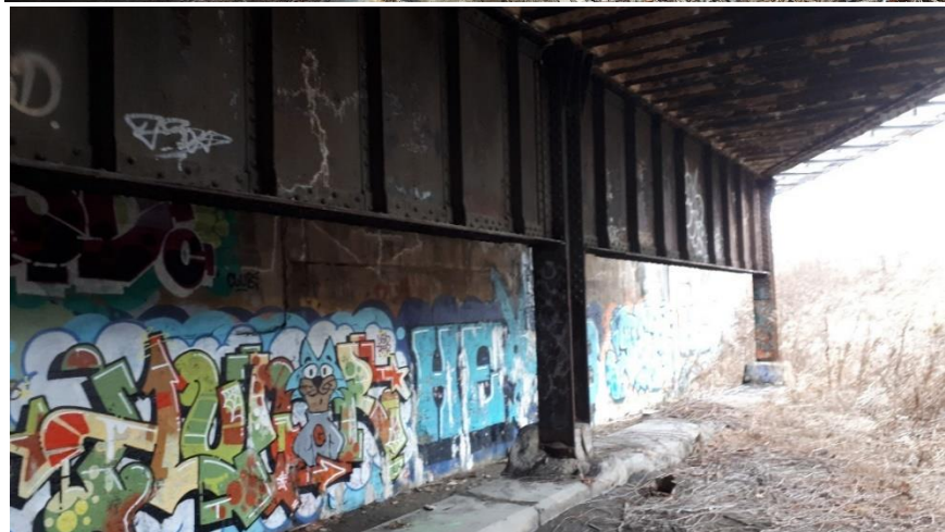
Plate 92: Detail of concrete pile footing.
