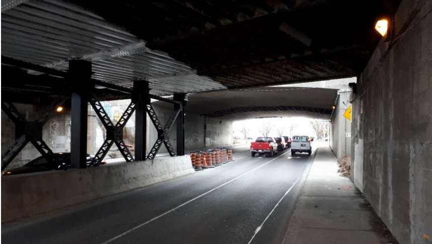
Plate 22: Concrete sidewalk and Parkside Drive on the western side, looking southeast.
