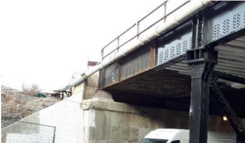
Plate 16: Detail of bridge bearings.
