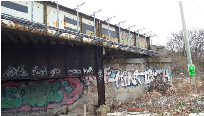
Plate 86: Western bridge abutment.
