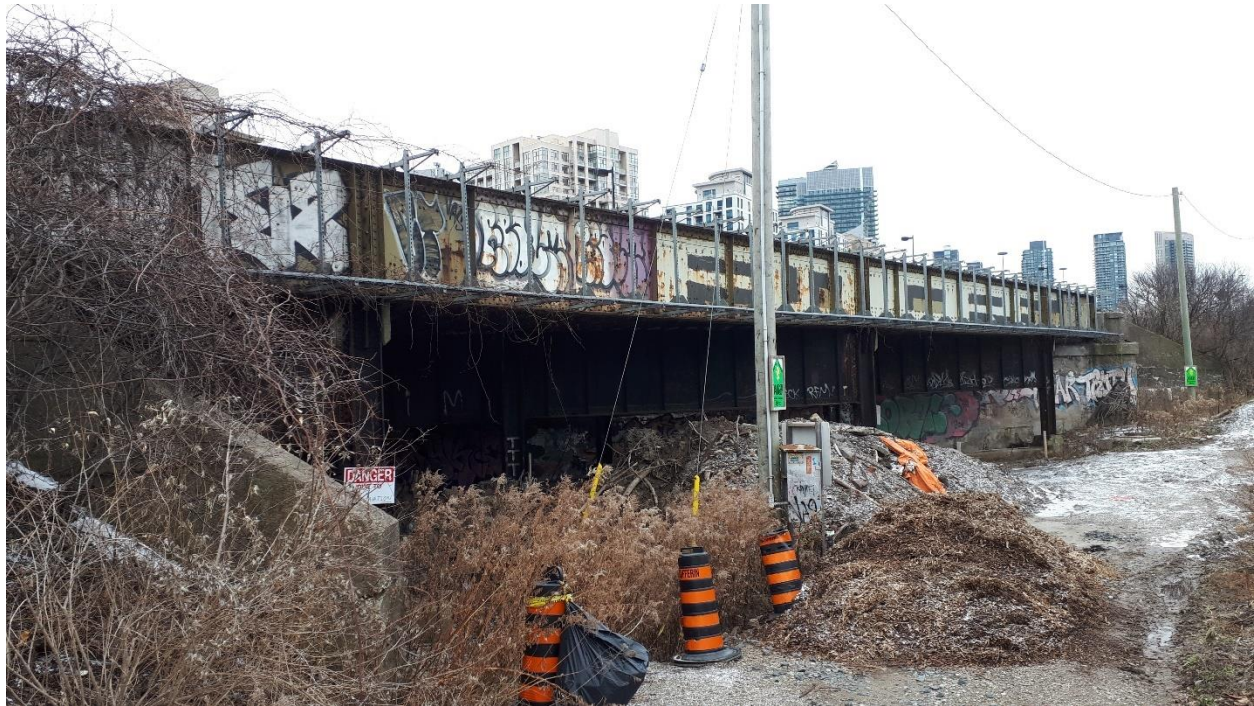
Figure 7: Former Queen Street Bridge (Mile 5.15), facing southwest.
