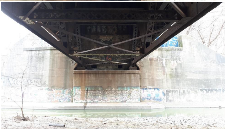
Plate 103: Detail of transverse, diagonal, and longitudinal steel beams, looking east.
