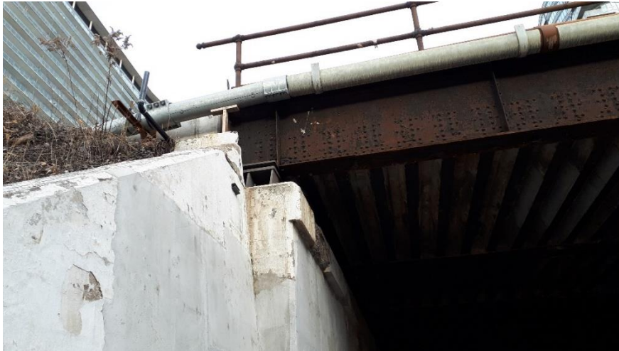
Plate 63: Detail of bridge bearing.
