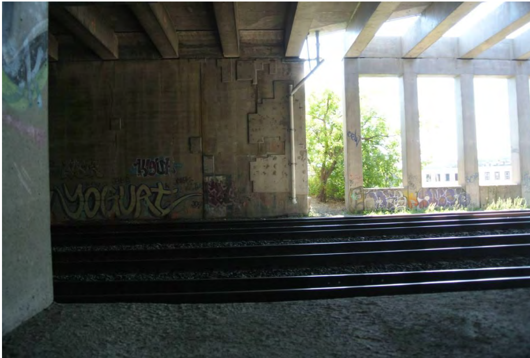
Figure 20: View towards southeast abutment, looking south.
