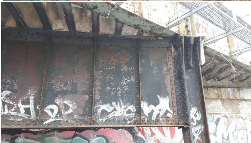
Plate 88: Detail of riveted connections.
