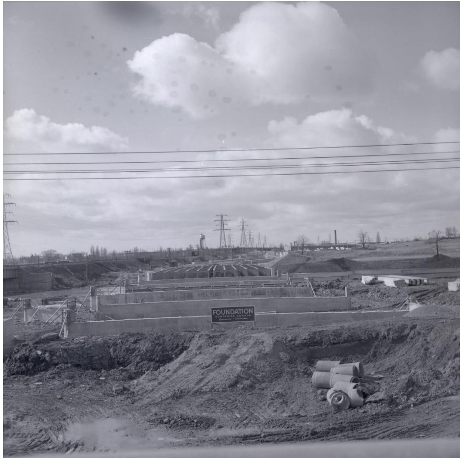
Figure 33: Photograph showing the Former Queen Street Bridge (Mile 5.15) in the left of the photograph (Salmon 1956b).
