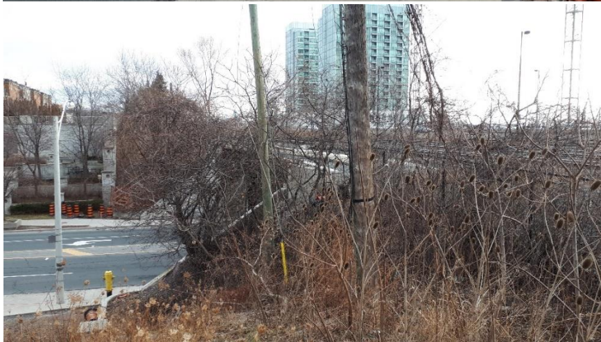
Plate 67: View of vegetation growth adjacent to the bridge.
