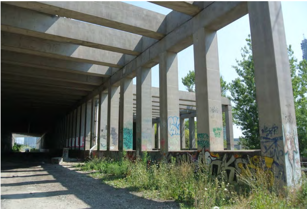
Figure 18: View toward west concrete columns, looking east.
