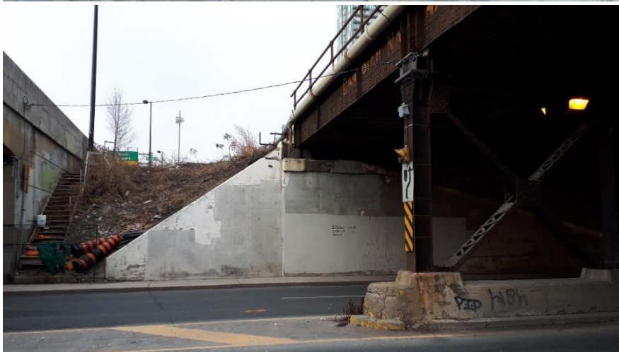
Plate 59: Western bridge abutment, looking west.
