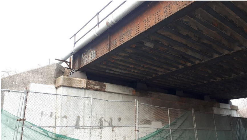
Plate 74: Detail of bearing and eastern abutment.
