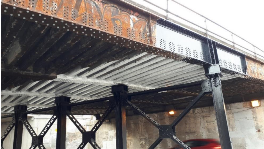
Plate 13: View of transverse and longitudinal beams and riveted connections.
