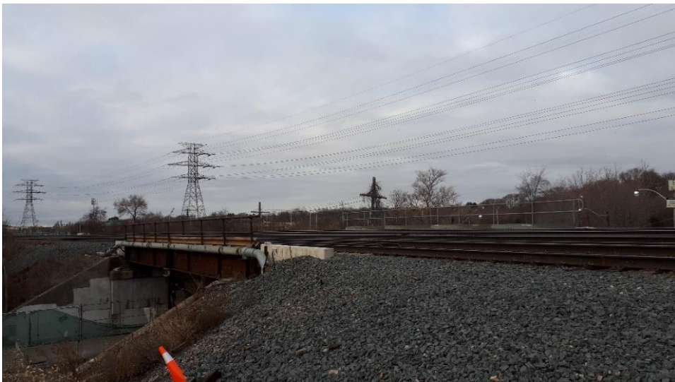
Plate 78: View of rail line over the Gardiner On-Ramp from Riverside Drive (Mile 4.90).
