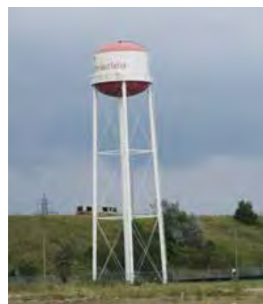
The Water Tower (ERA 2019).
