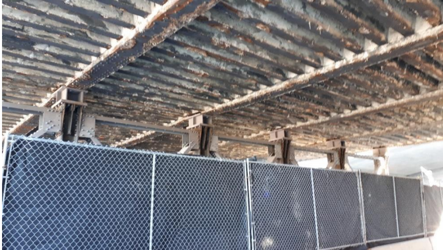
Plate 49: Detail of bearings on top of “X” bracing.
