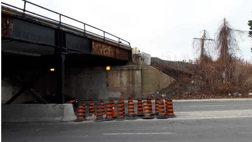
Plate 10: Western bridge abutment, looking west.
