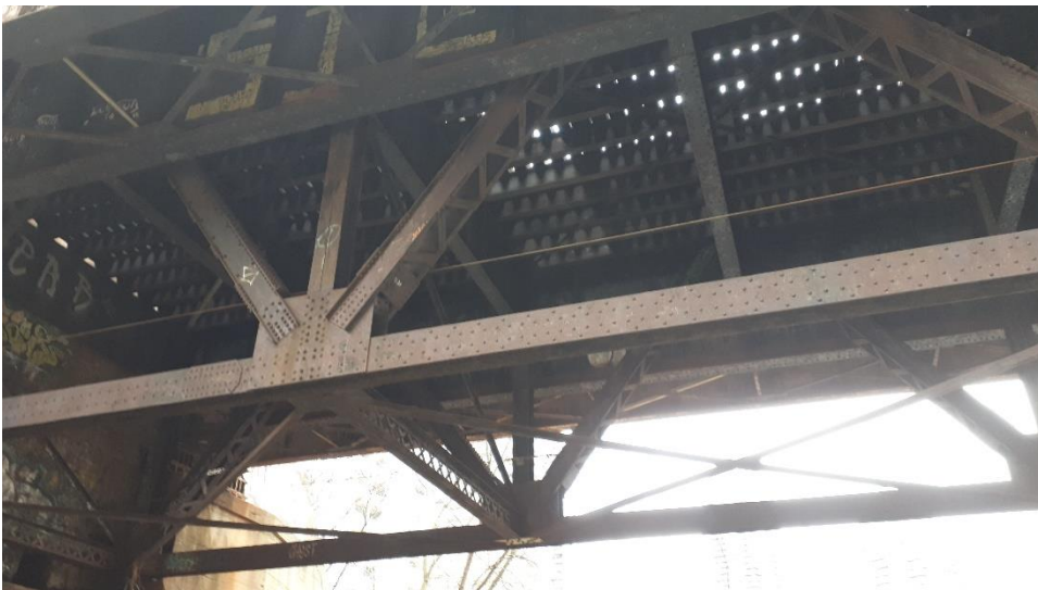
Plate 105: Detail of deck truss and bridge soffit.
