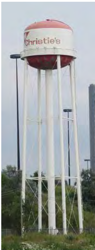
Water Tower (ERA 2019).
