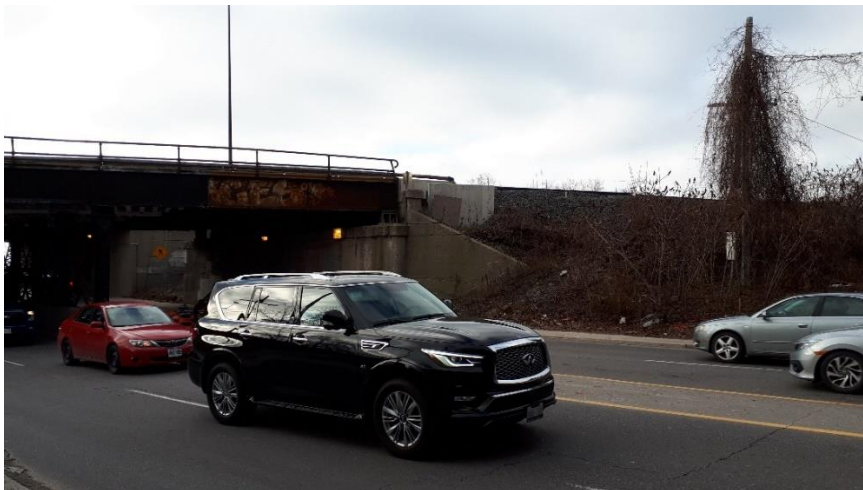
Plate 3: Western bridge abutment, looking southwest.
