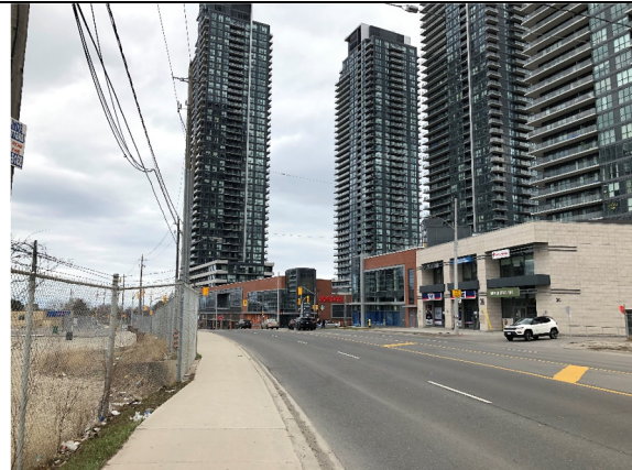
Plate 2: View south toward condominium towers on west side of Park Lawn Road.
