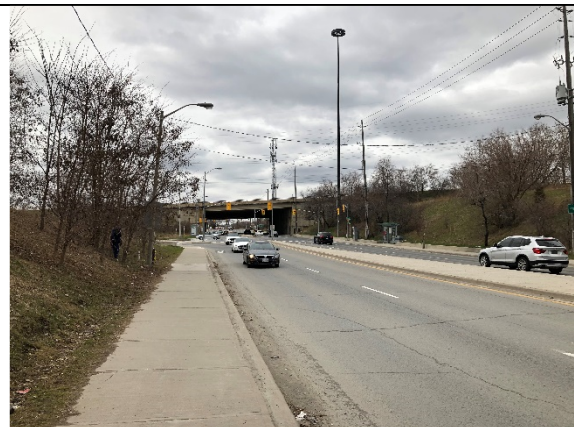
Plate 6: View looking north to expressway along Park Lawn Road from the rail corridor.
