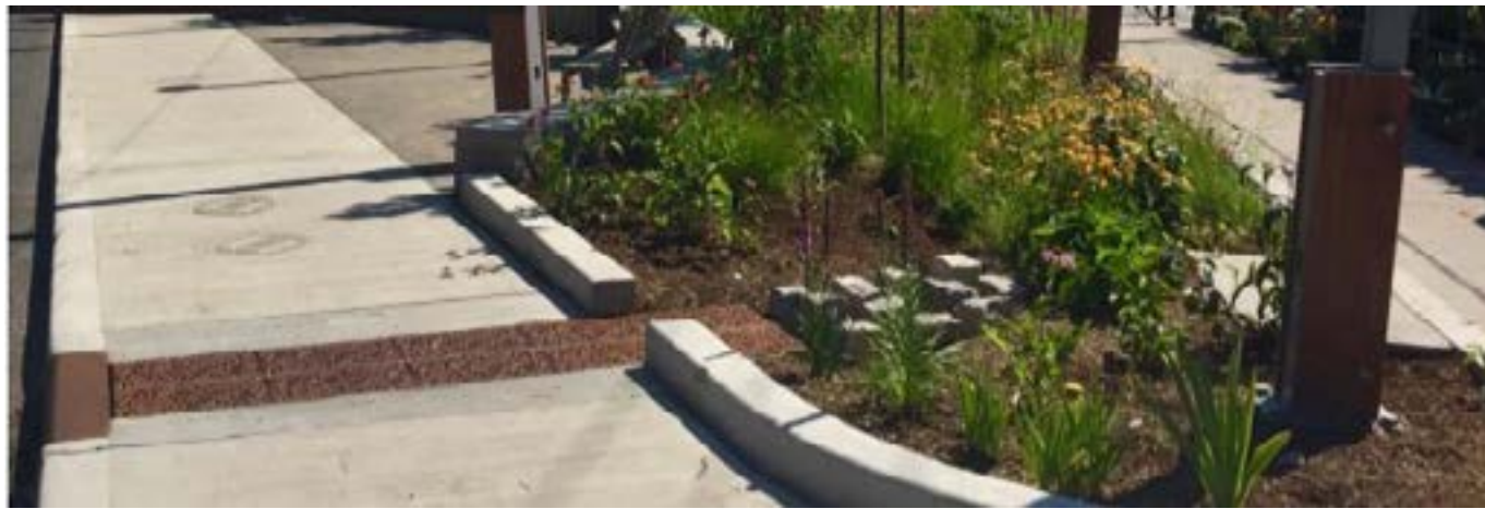
Figure 6 - Conveying flows to tree pits/rain gardens
